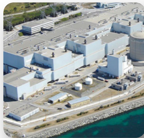
Darlington Retube & Feeder Replacement Project
