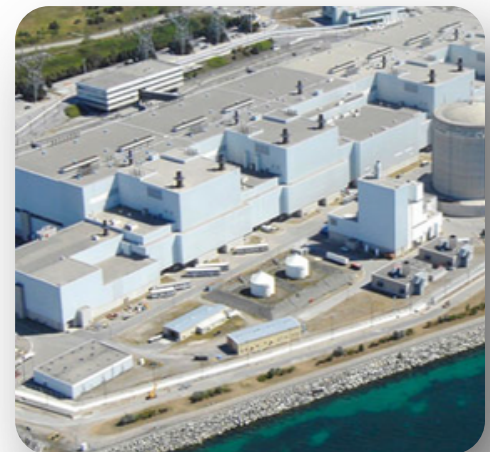
Darlington Retube & Feeder Replacement Project
